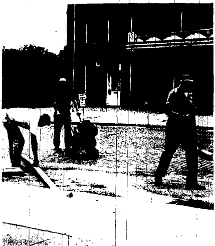
PAINTING PARKING STALL LINES downtown Sunday were, from left, Street Commissioner Vern Schulz, Gerald Otte behind the painting equipment and Leonard Schwanke. Alvin Geher was also a part of the crew but is out of the picture to the right. Schulz and his crew used approximately 20 gallons of white and yellow paint getting all of the parking stalls painted Sunday and Tuesday. A breakdown in the painting equipment prohibited them from getting the job finished Monday.
